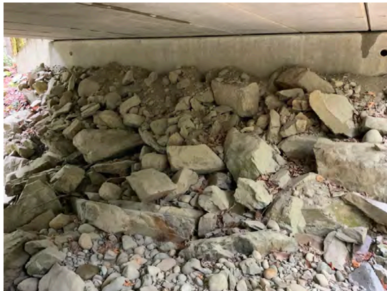
Right Bank Abutment when facing downstream
