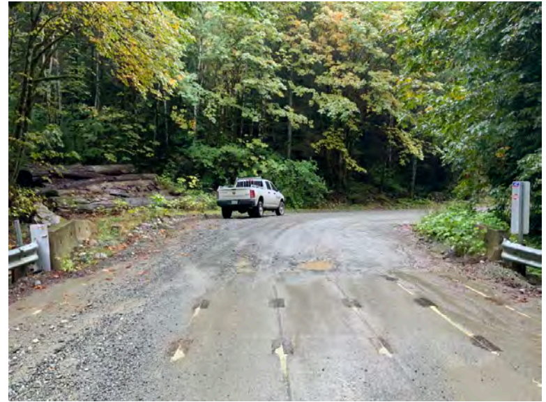
Approach from Left Bank when facing downstream
