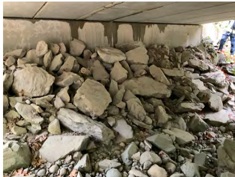
Left Bank Abutment when facing downstream
